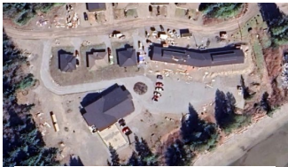
image a) - Project Location 1
