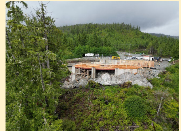
Government Building Progress, June 2025
