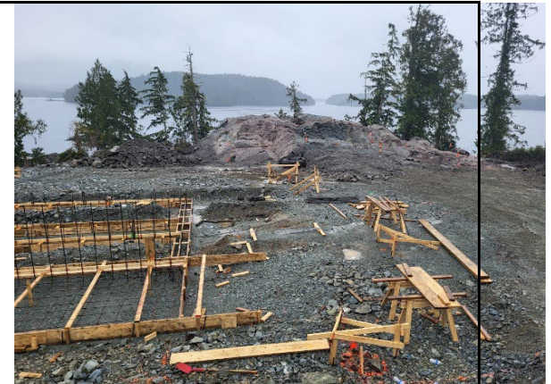
Government Building Progress, March 2025
