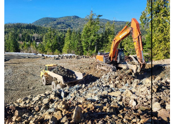
Phase 2 bulk cut and fill in progress
