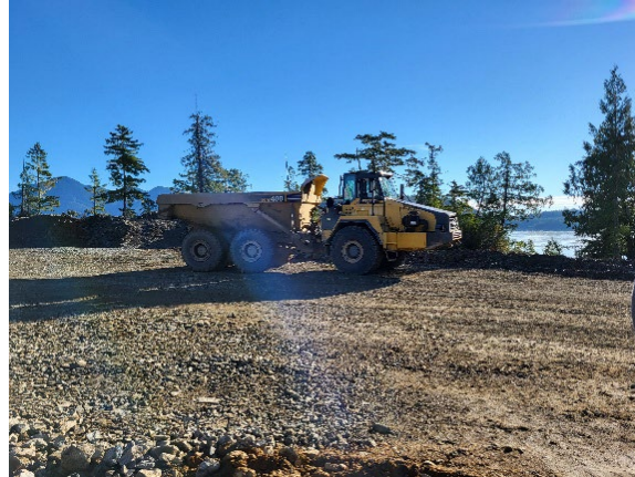
Phase 2 bulk cut and fill in progress, Dec 2024
