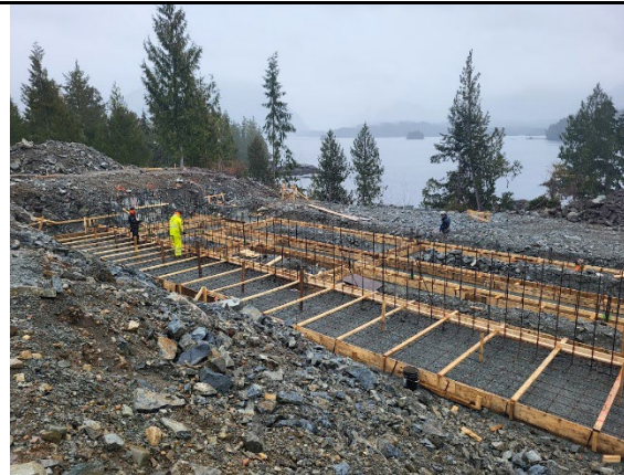
Government Building Progress, March 2025
