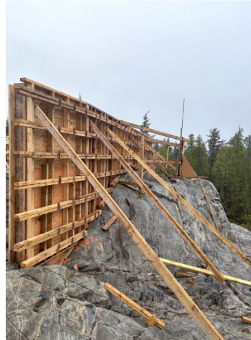
Government Building Progress, March 2025
