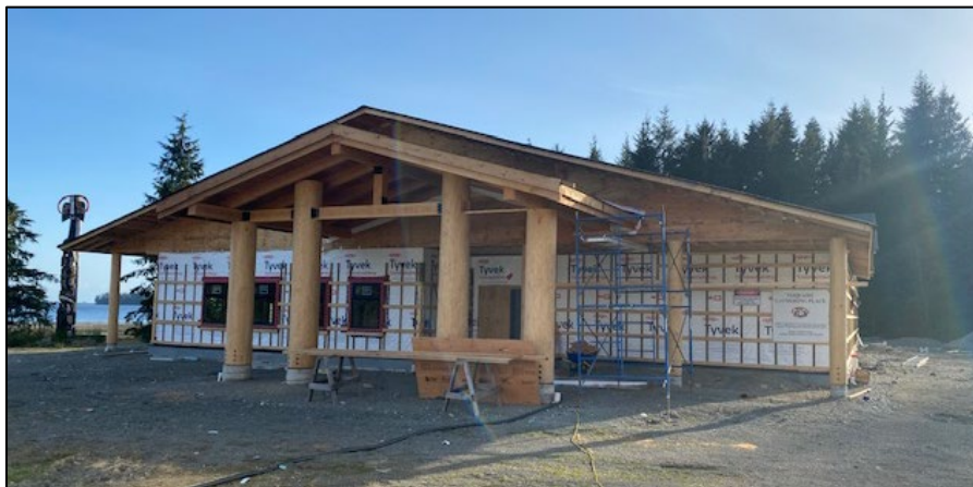
Community Building exterior progress, Spring 2021
