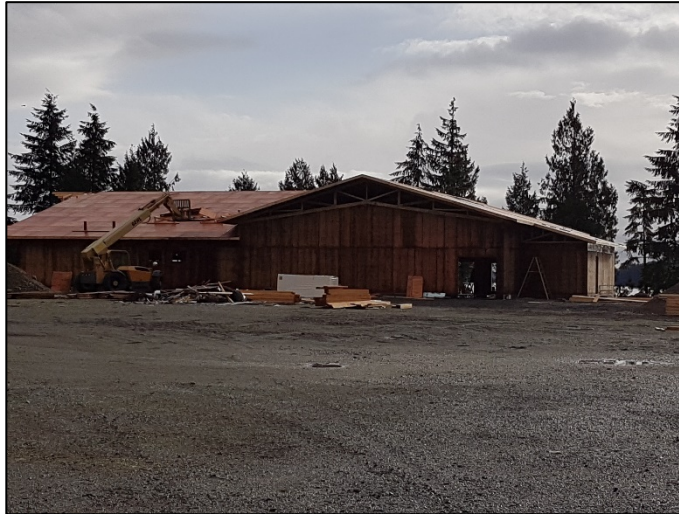
Roofing installation on Community Building
