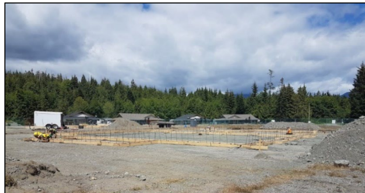
Excavation complete; footings and re-bar being installed
